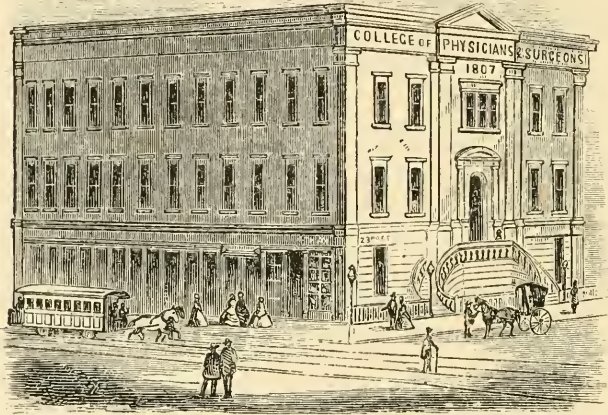
THE COLLEGE BUILDING IN TWENTY-THIRD STREET.
